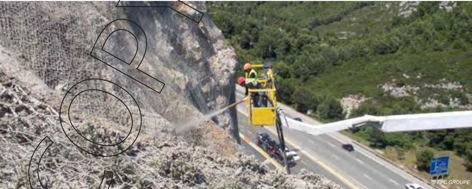
Technicians are spraying fiber concrete in order to protect the more weathered areas. A 100 meter crane was used.
